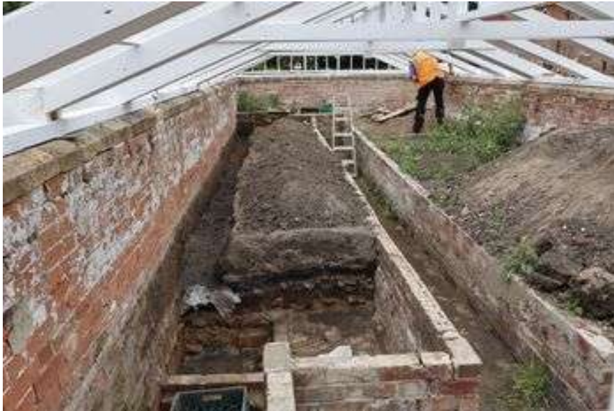
Clearing the sunken greenhouse
