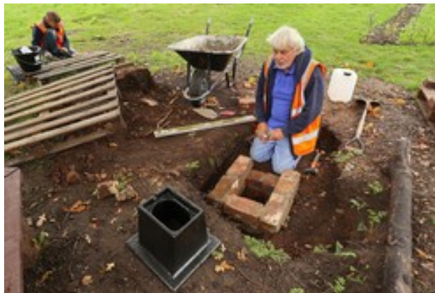
Alan finishing Victorian water valve.
