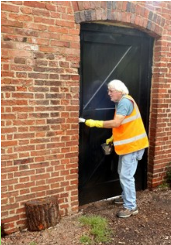
Alan , giving a final acid wash to the repaired west wall door
