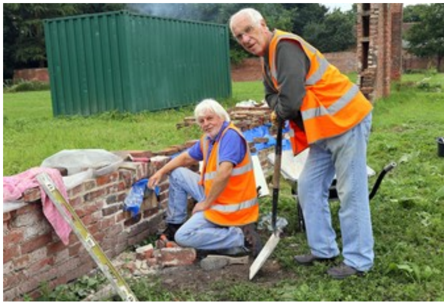
David and Alan working on the central wall
