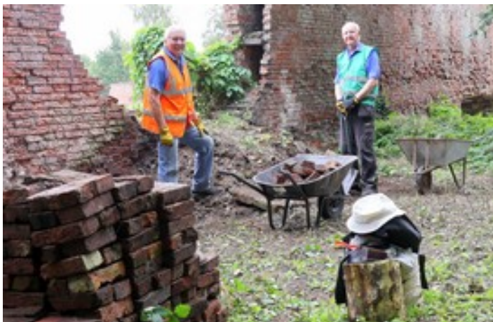
Russ and Ralph working on south wall
