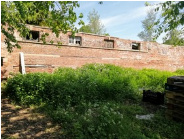
North wall 'accommodation'
