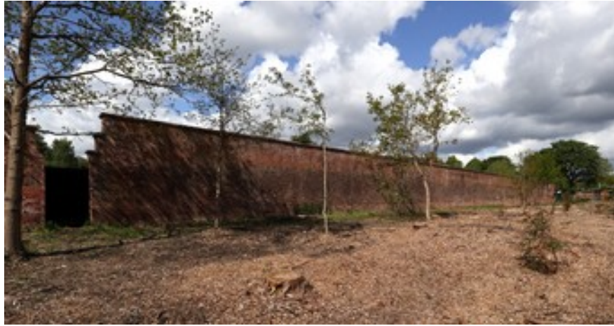
East slips cleared of trees
