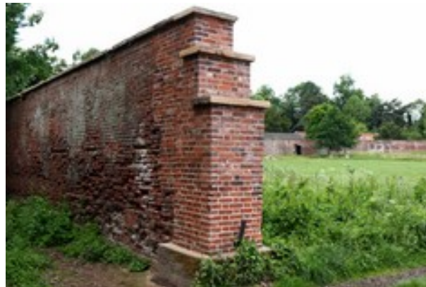
South wall gate repaired
