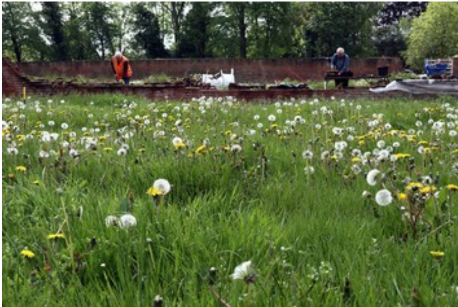
Central wall conservation
