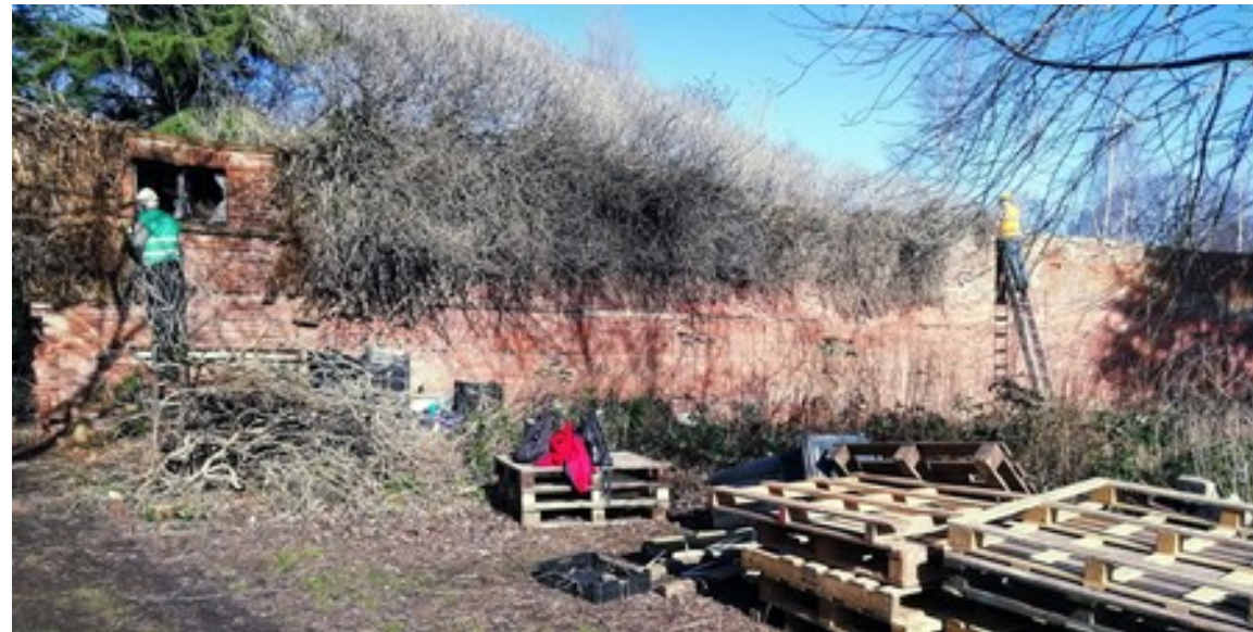
Clearing the north wall
