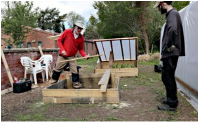
Robert and Brian building the cold frames
