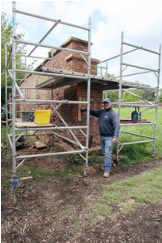
South gate repairs by Bonsers
