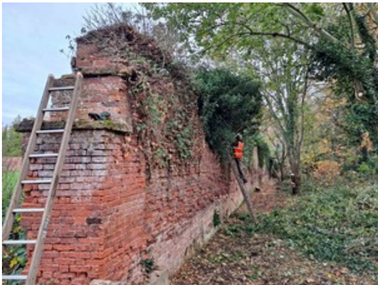
Clearing south wall prior to restoration
