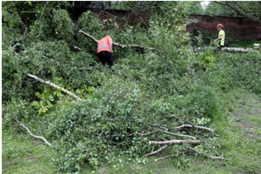
Tree clearance next to west wall
