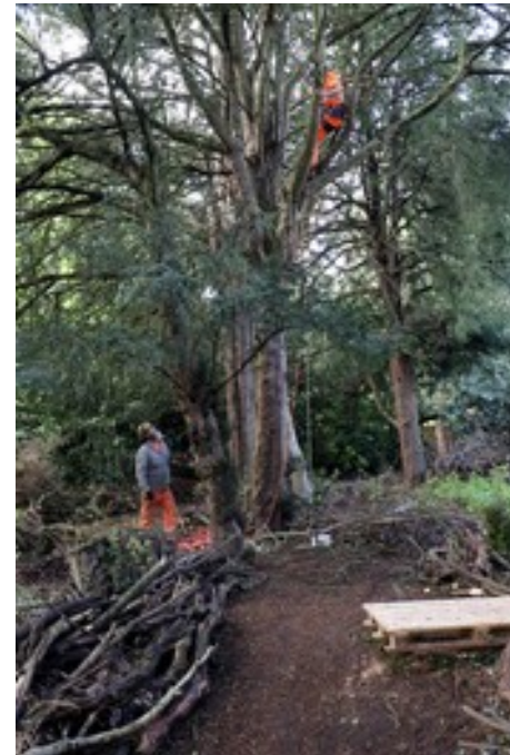
Trimming trees near cottage
