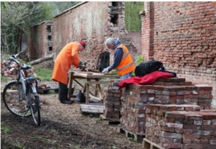
Ralph and Russ preparing bricks for south wall repairs
