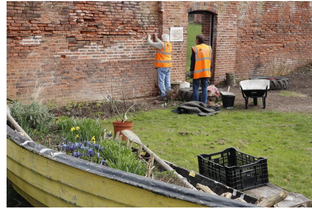
Alan and Andy repairing the wall
