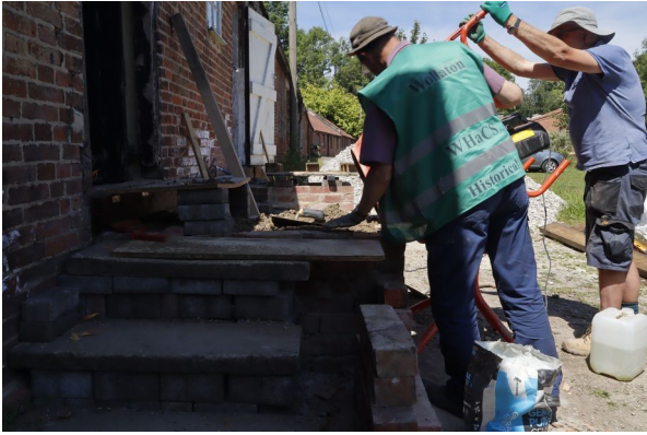
Peter and Geoff working on the access ramp
