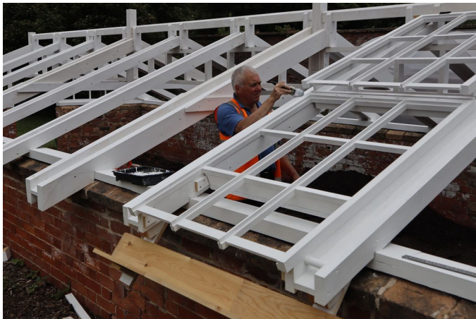
Test frames, giving an idea of the finished roof
