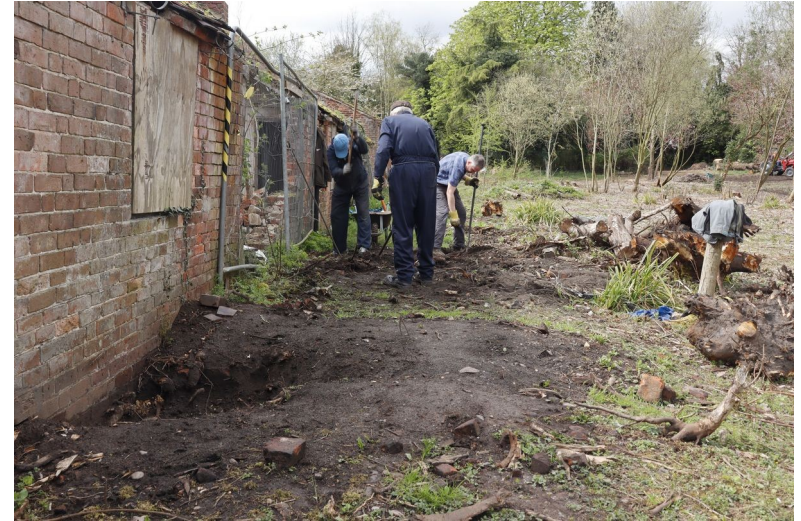
Clearing more roots and rubble from north slip garden
