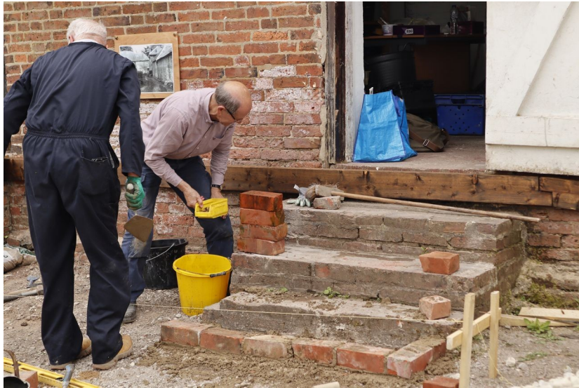
More work on the access ramp
